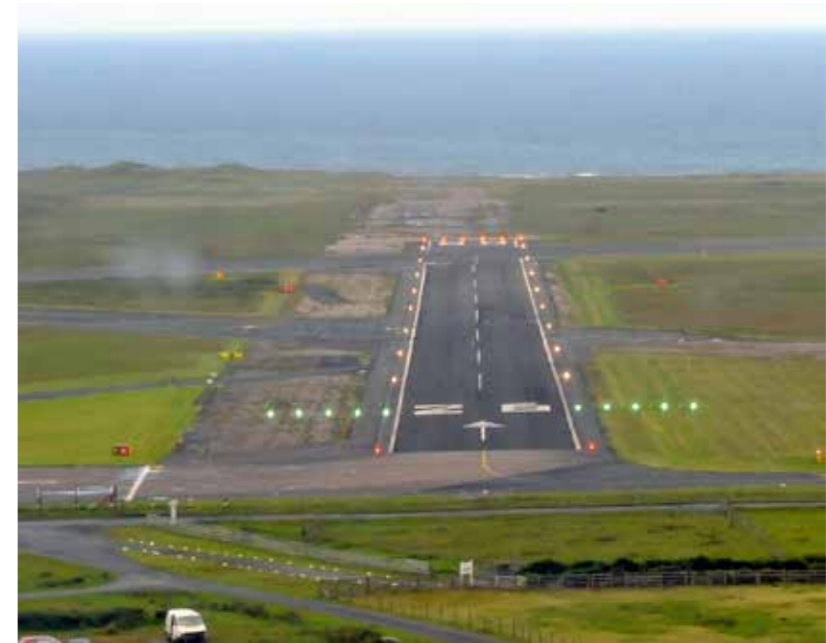
Final approach to Islay's Runway 08/26 which has been reduced in length to 2,083ft (635m) – the original length and width of the former RAF Port Ellen air strip is still evident as the Islander comes in to land from the east.
